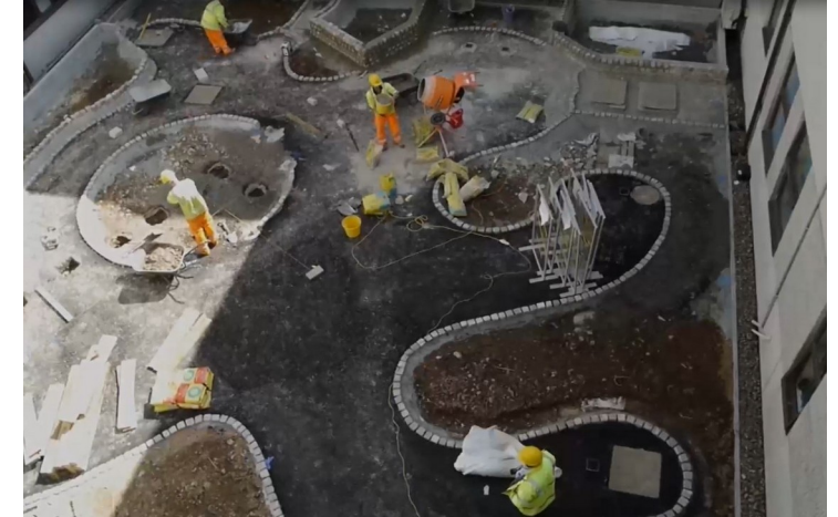
Construction: Reuse of granite materials enhancing visual quality. Credit: Cormac Solutions Ltd
