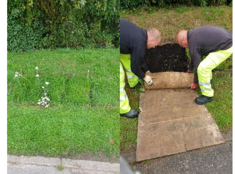
Wildflower turf installation on a bank at Campdowns Cemetery, Carlyon Bay, Cormac
