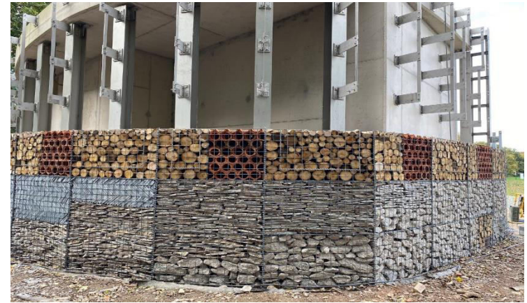
The external wall during construction – showcasing the gabion sections Credit: Thames Tideway
