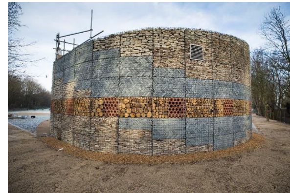
The Kiosk comprising of mixed materials to form various habitats for wildlife
