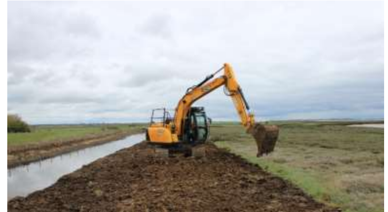
Removal of the south-east embankment through the process of managed realignment to create new saltmarsh © Katherine Gilchrist
