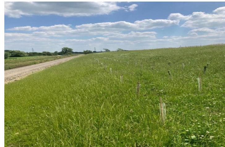
Grassland meadow post-seeding works (railway embankment)
