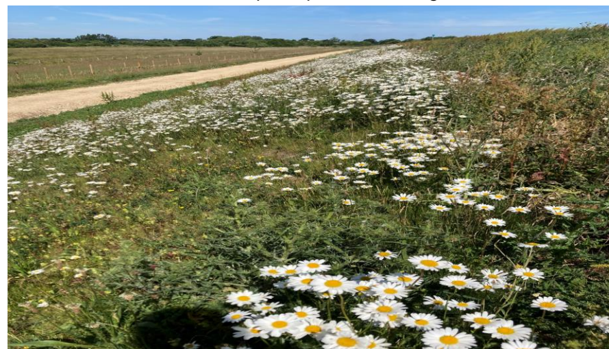
Post seeding works (Railway embankment)
