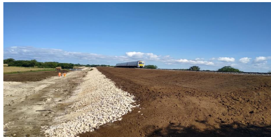
Installation of topsoil, prior to seeding works
