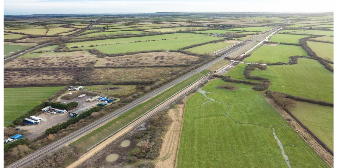
Drone image during construction, 2022 (Mulholland)
