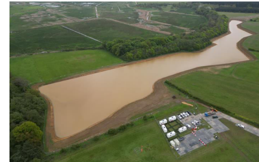
Aerial view of the wetland
