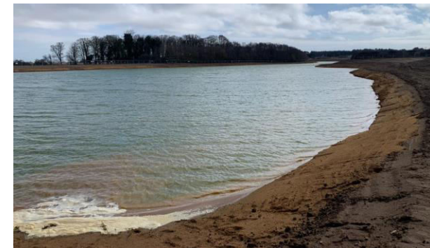
The newly created wetland edge prior to planting
