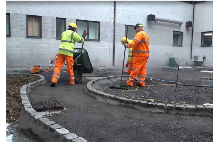
Cormac on site during construction Photo Credit: Cormac
