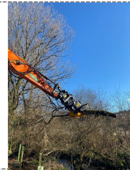
Clearing the riverbank
