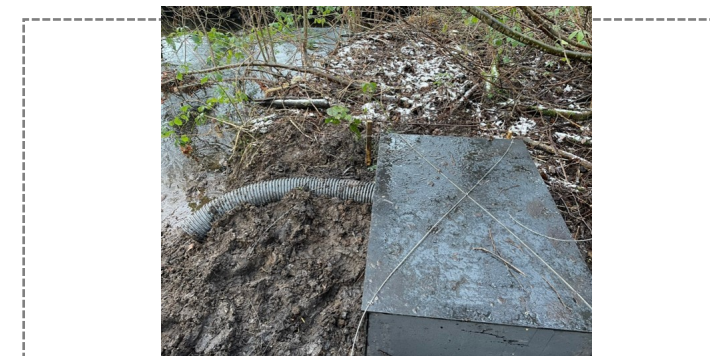
Process of installing artificial otter holt at riverbank
