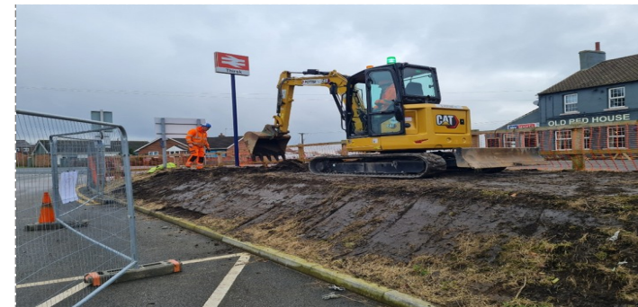
Reprofiling of embankment prior to seeding and planting.
