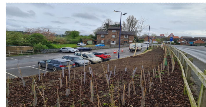
New planting and wildflower seeding on embankment.
