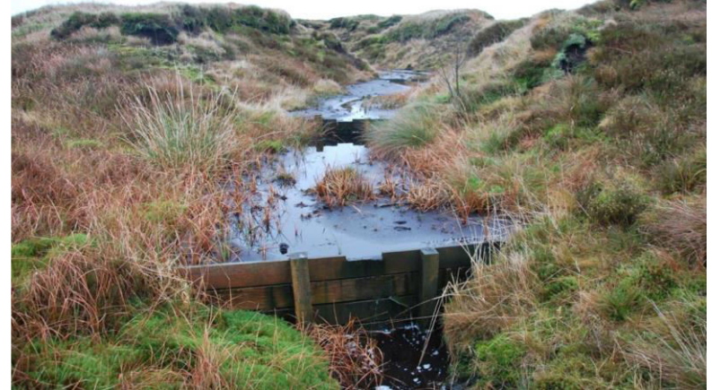
Close up of timber dams & water retention used in Peatland Restoration
