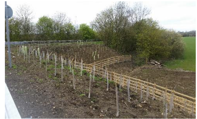
Embankment North side – 2 weeks following landscaping works
