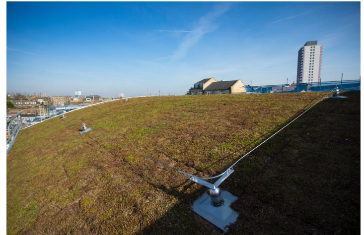
Green Roof at Eleanor Street Site. Taken by John Zammit.
