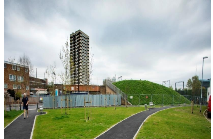
Green Roof at Mile End Site. Taken by John Zammit.
