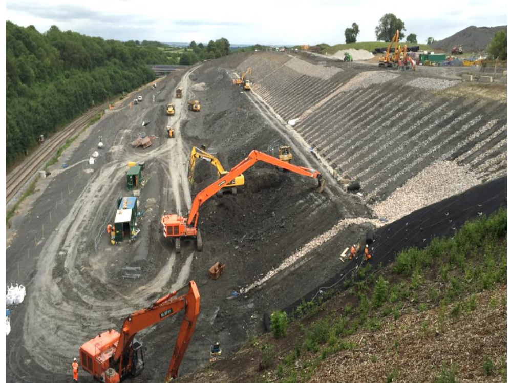
Re-grading Railway Cutting
