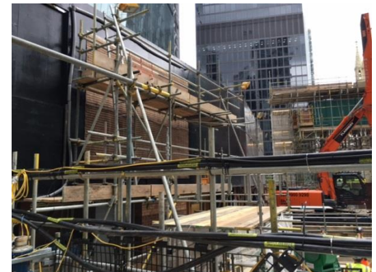
Under construction day 3
