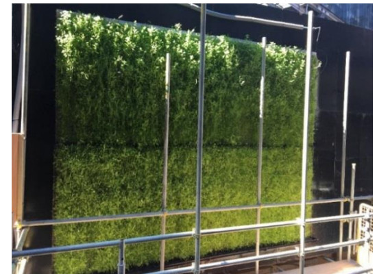
Living hoarding progress, day 26
