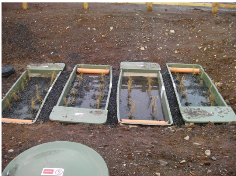
Photo: Reed beds for site office waste disposal
