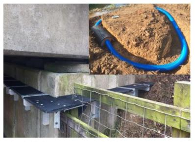
Otter holt habitat improvements included creation of new artificial holts and an otter ledge over the River Avon; both constructed from recycled site materials
